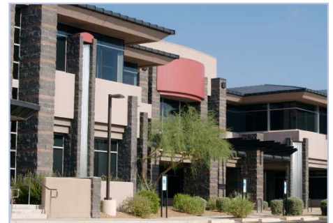
Vegetation too close to windows.
