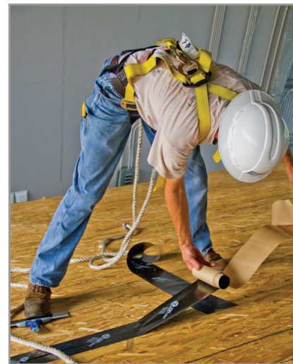
Sealing the roof deck.
